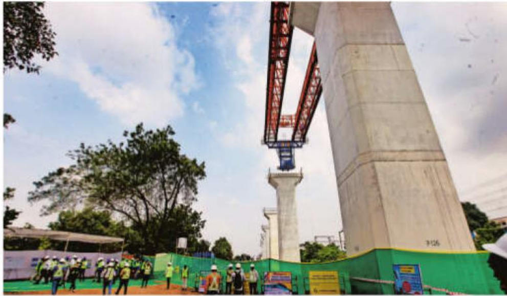
Construction underway for the project in Vadodara city. Bhupendra Rana
